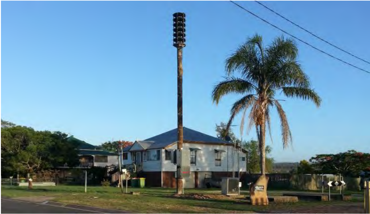
EMALTE designed and installed system at Grantham, QLD, Australia
