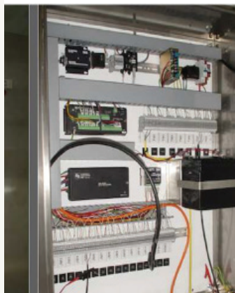
Automatic Pore Pressure Recording System AL-131-VWP
